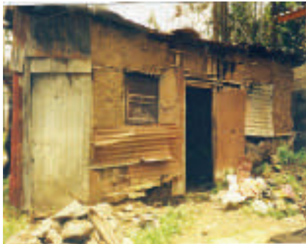
"This is the house for the family"!
